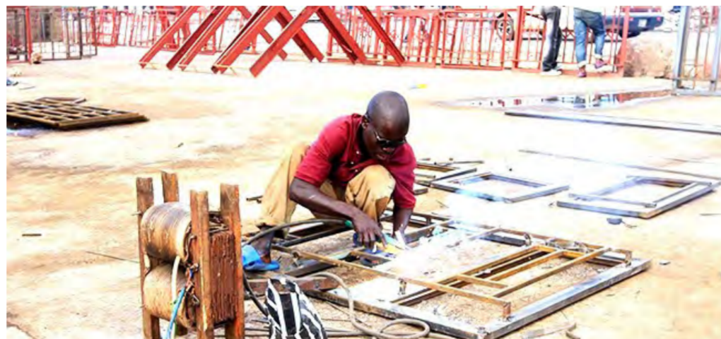
A WELDER on duty at a workshop in Garden Township.
